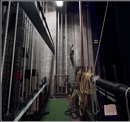
Above the stage: fly floor.
